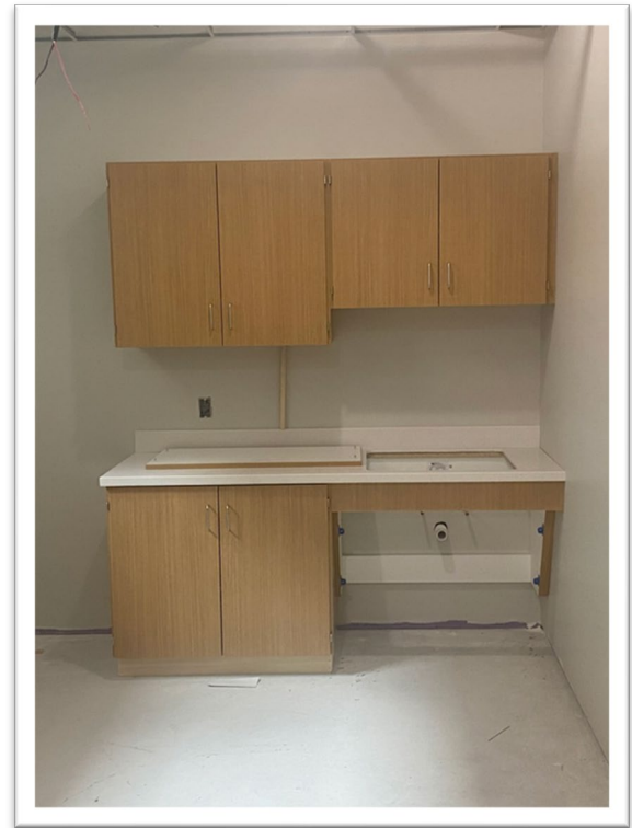
Casework installation in the health room has begun.
