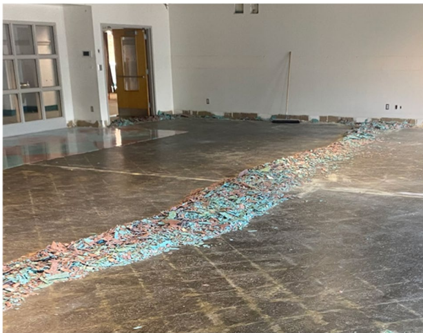
Completing flooring demolition in the cafeteria.
