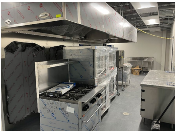
Kitchen equipment installation has started.
